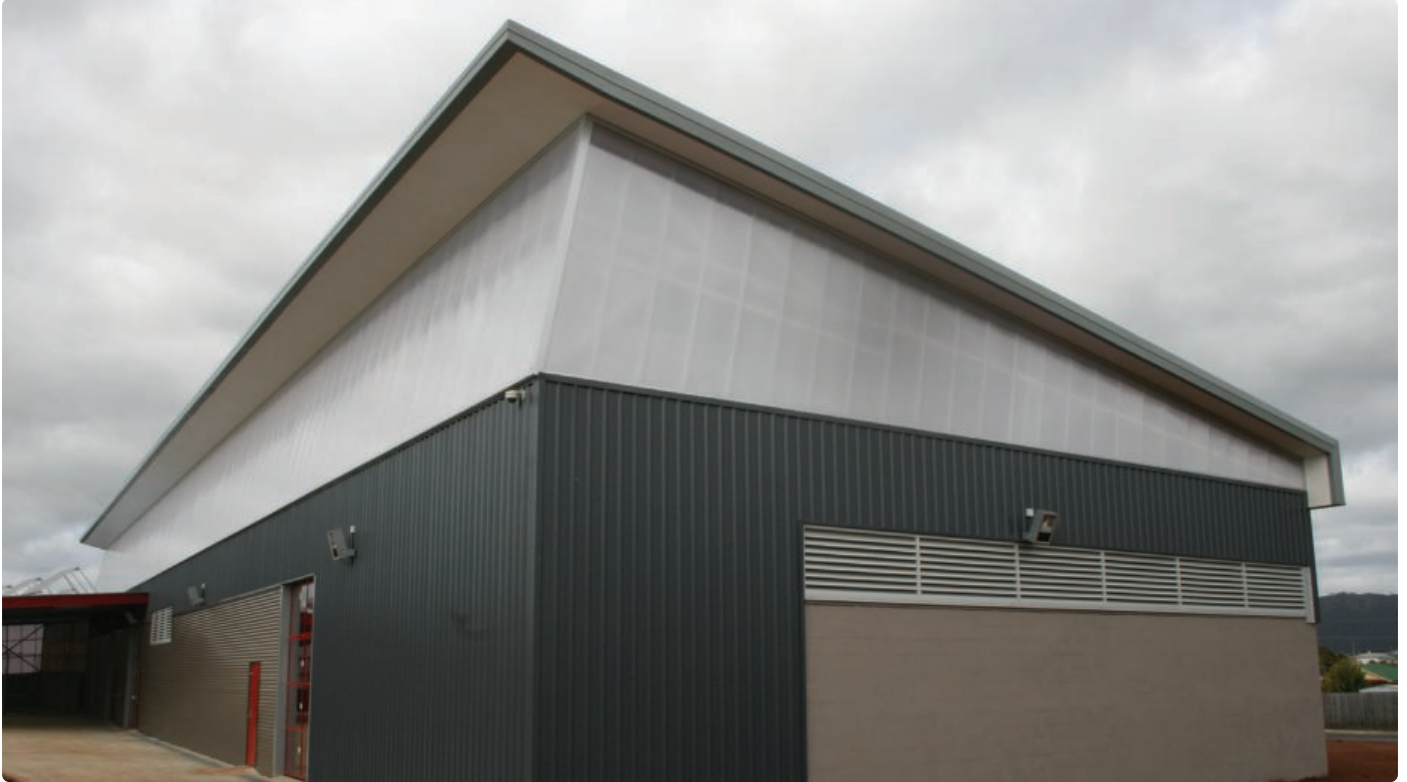
George Town Trade Centre Tasmania, Australia | Architect: Loop | Application: Sidelight | SUNPAL® Type: White Ice 10mm
