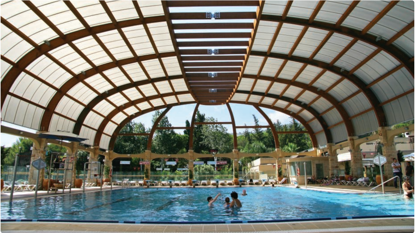
Sports Complex at the Technion Institute of Technology, Israel | Application: Roof - 3,200sqm | SUNPAL® Type: 18mm Diffuser Plus Bronze
