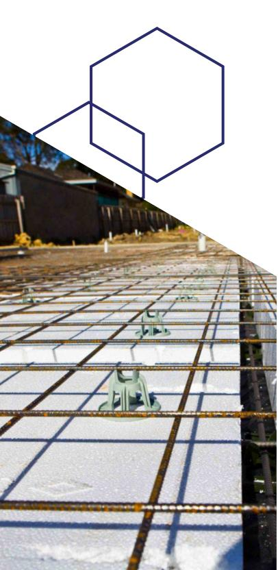
StyroPod by Foamex is an Australian made, lightweight EPS waffle pod void former perfect for use in concrete slabs in the building and construction industry. Designed specifically for use in residential building, StyroPod (formerly known as Diamond Pod) waffle pods provide under slab insulation and support, working in unison with natural soil movements, and lowering the amount of concrete required for a build.
